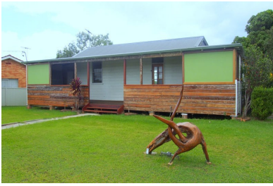
15 High Street, Urunga 'MAJOR RENOVATIONS'
